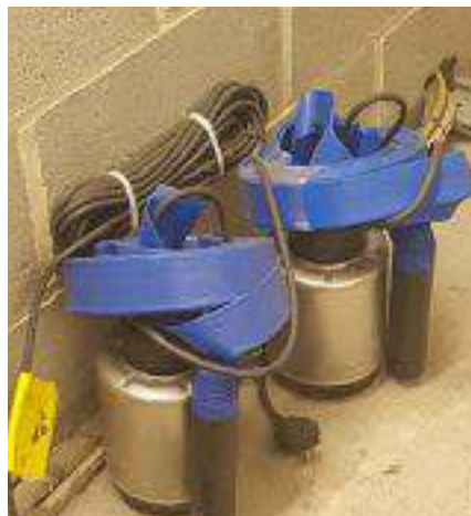
2 puddle pumps to help with the removal of water.
