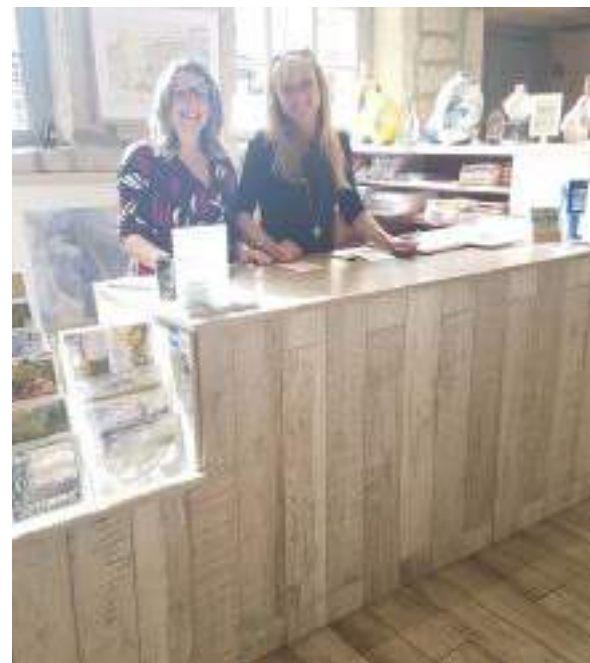
Counter base and new shelving is made from marine ply and coated with sealant.
