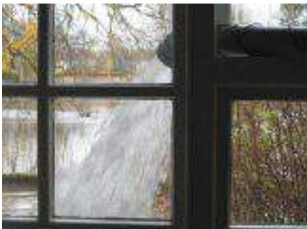
Pumping water out through the window.
