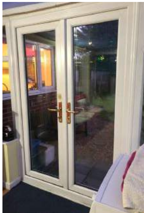
Flood resilient patio doors have been installed.
