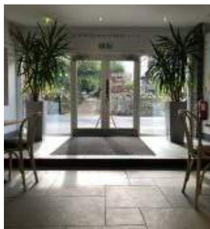
The tiled and tanked walkway through the hotel.
