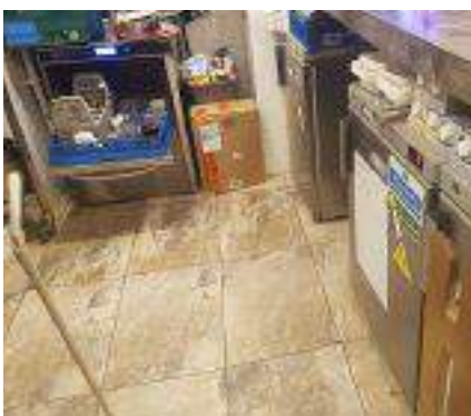
Tiled kitchen floor with waterproof adhesive and grout.
