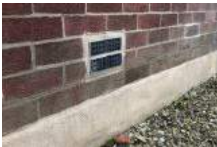
Self-closing air bricks and waterproof rendering was applied underground to the foundations and 30cm (12") above ground.
