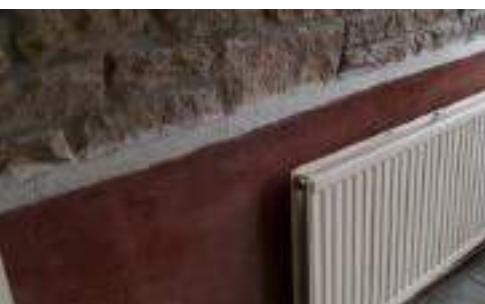
The walls were rendered on top of the membrane, using coloured renders
