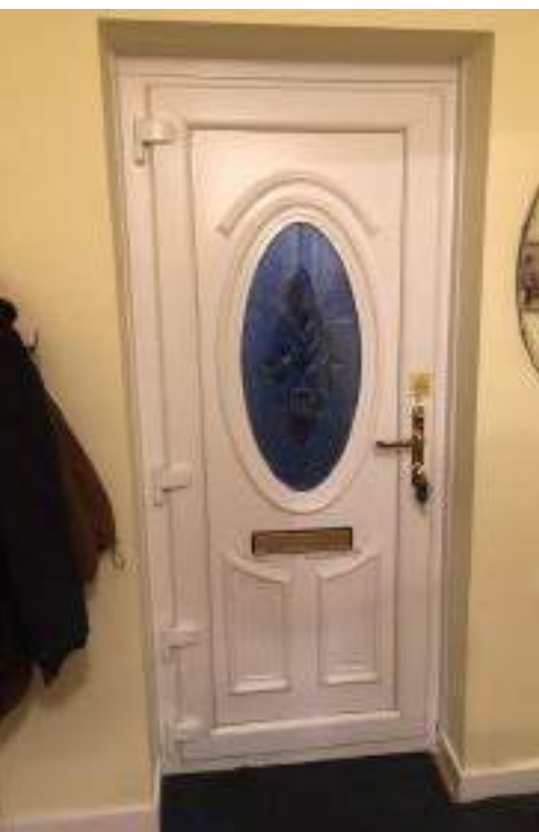
Flood resilient front door has been installed.
