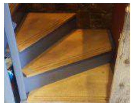
Steel staircase and solid oak treads.
