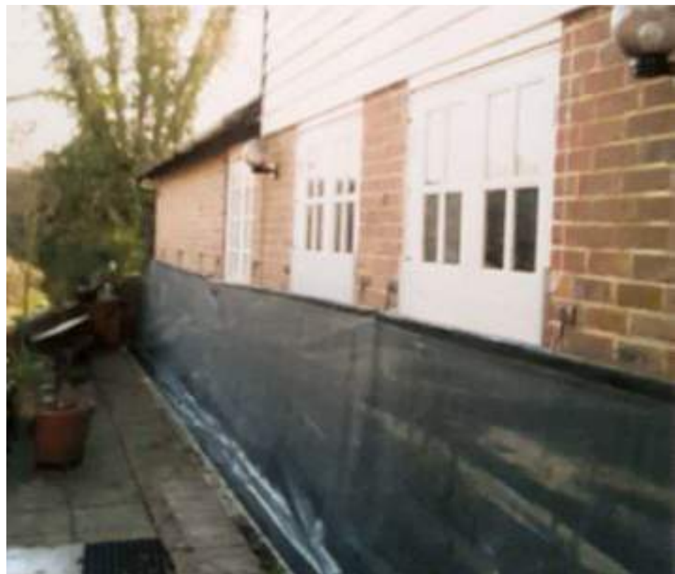
The building skirt system can be pulled up to around a metre high round the whole house when needed.
