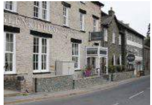
A robust flood wall around the front and river side of the hotel, into which demountable flood barriers are fitted.
