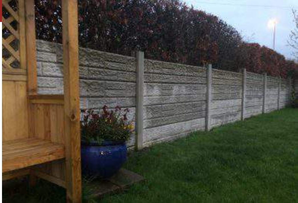
A 'concrete type' fence has been erected to hopefully slow the flow of water, providing extra time to evacuate.
