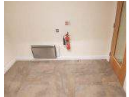
The lower section of the wall was re-plastered using a breathable renovating plaster.
