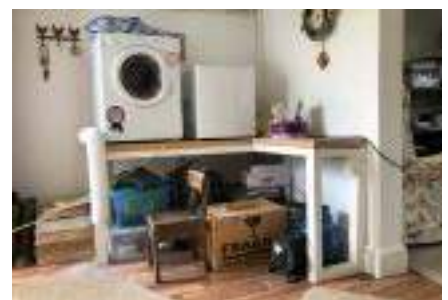
White goods in the utility room are now on a plinth and even the wood burning stove in the lounge is raised up.
