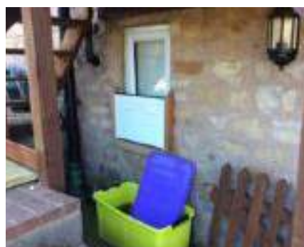
Flood barrier to basement door and window.
