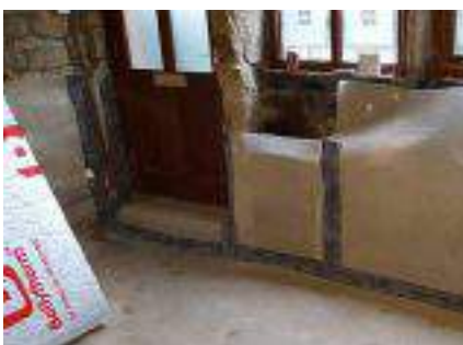
Waterproof membrane during installation.
