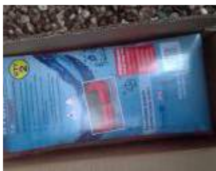
Absorbent packs swell up and block water.
