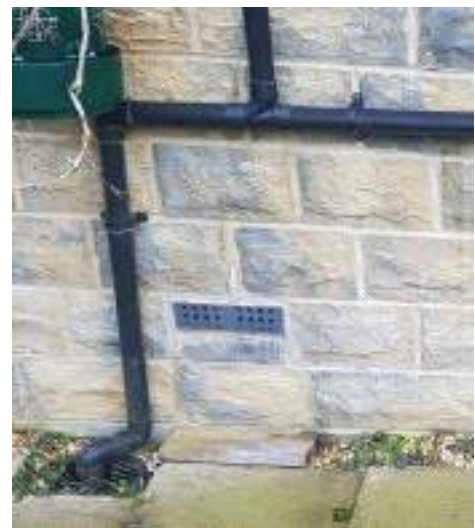
Waterproof render onto the bricks and self-closing airbricks.
