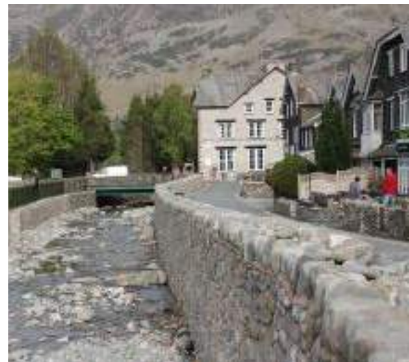
Newly upgraded Environment Agency defences.
