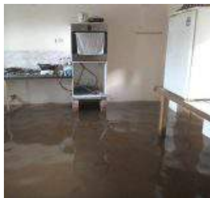
The kitchen during the flood of 2020.
