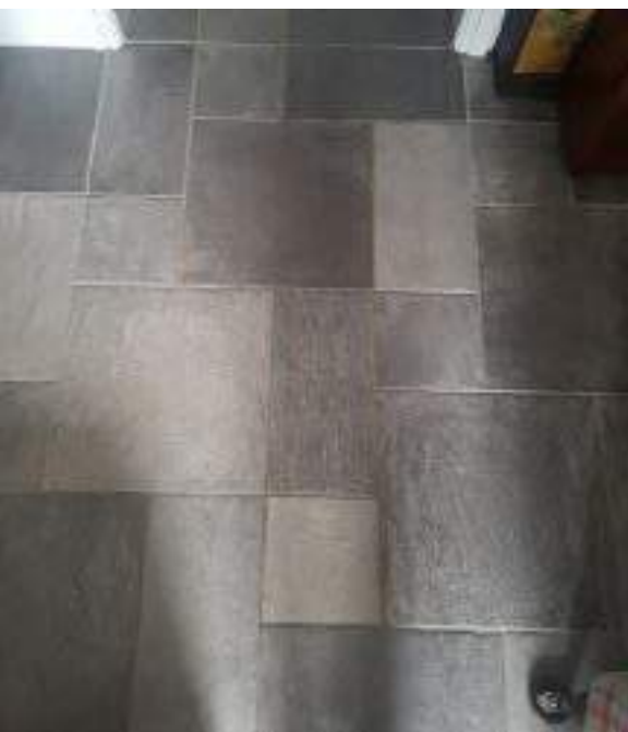
Tiling in the ground floor above insulation and underfloor heating.
