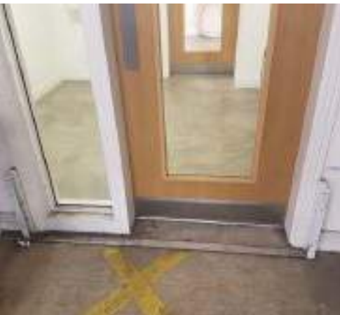
Flood barriers to all doors and UPVC door architraves.
