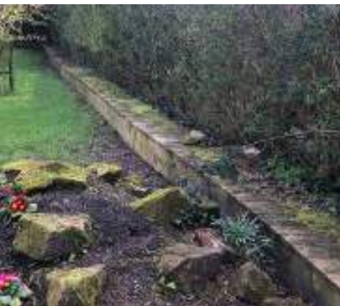
Wall with substantial foundations in the garden.
