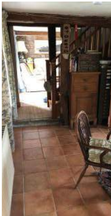
Floor is tiled, enabling them to just sweep the flood water out of the doors.
