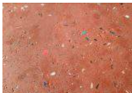
The walls were rendered using coloured renders.
