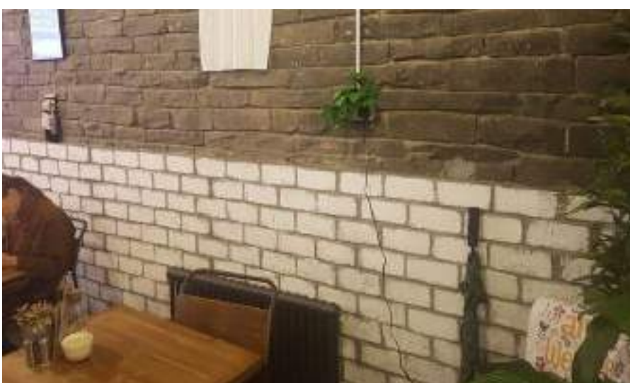
Walls stencilled and painted to resemble tiling.
