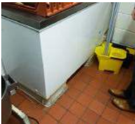
Some kitchen equipment is sited on crates.
