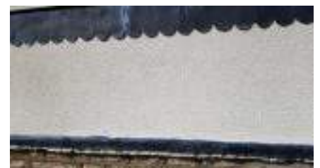
Walls on river-facing side of house have multi-layered waterproofing.
