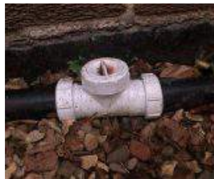
Non-return valve in pipework, to prevent backflow.
