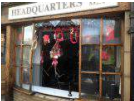
The pressure of the flood water inside caused the windows to blow outwards when the flood receded.
