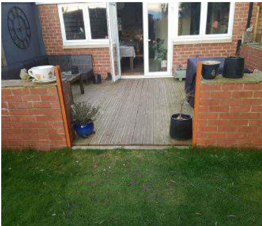
A flood wall has a flood-proof gate for access to the patio area.
