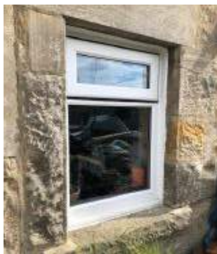
Original window replaced with a flood proof window.
