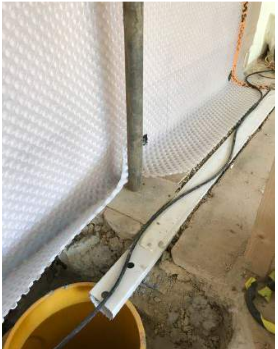
Cavity drainage membrane system and sump pump during installation.
