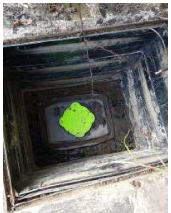
The culvert running underneath the house now has two non-return valves.
