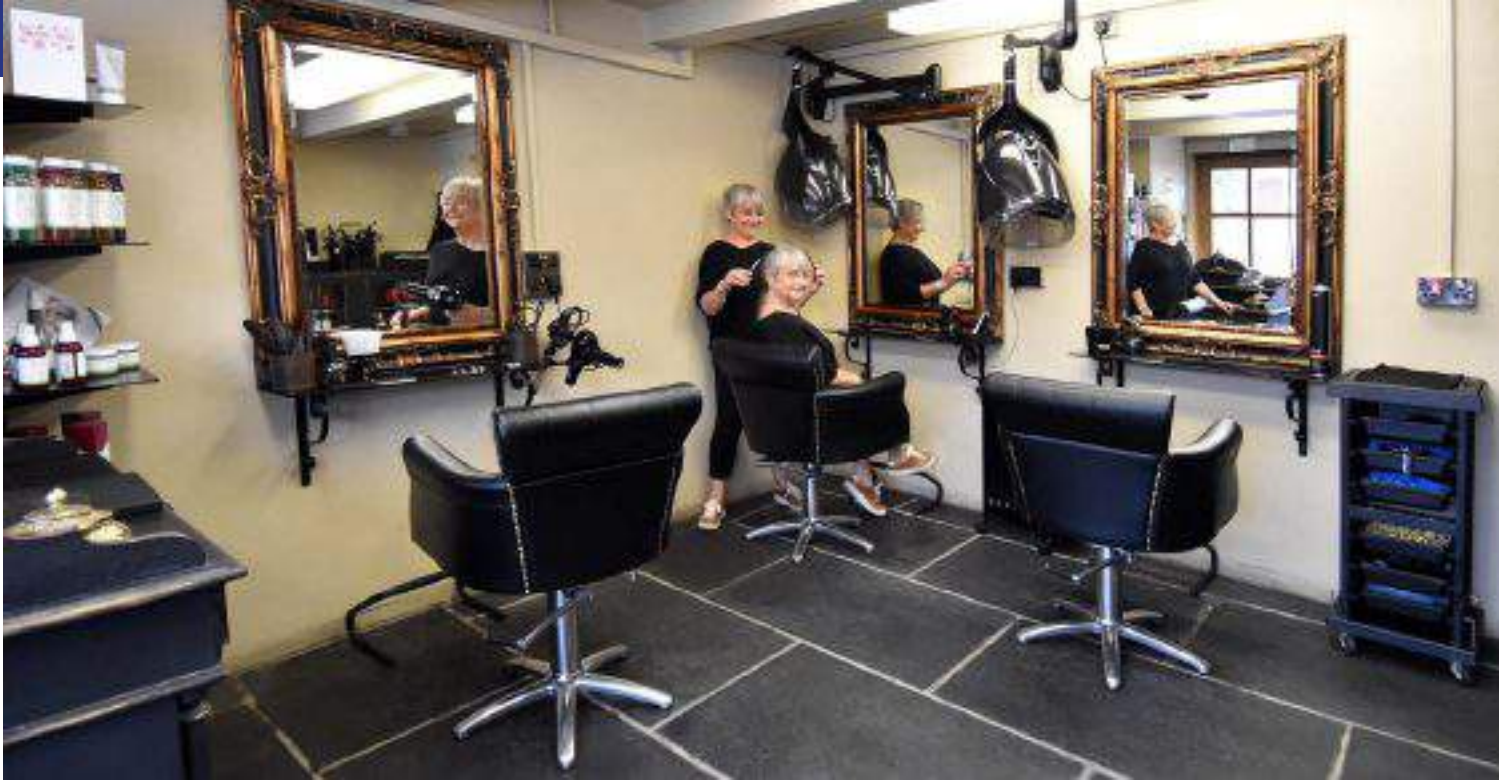
Stone flagged floor and the walls have a plastic membrane from floor to ceiling, with cement render over the top.
