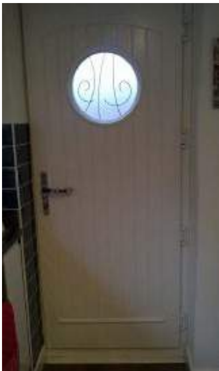
Flood resilient doors have been installed.
