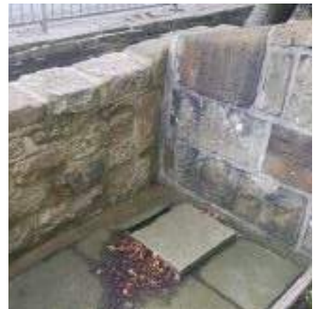
Sump created, into which powerful submersible pump can be dropped when flooding commences.
