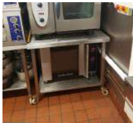
Kitchen equipment is on wheels and can be moved easily.
