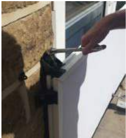
Fitting new taller but lightweight barriers.
