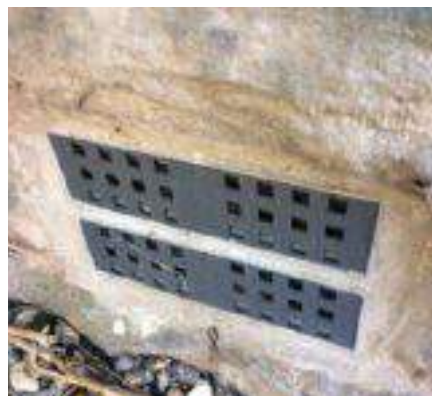
Self-closing airbricks.
