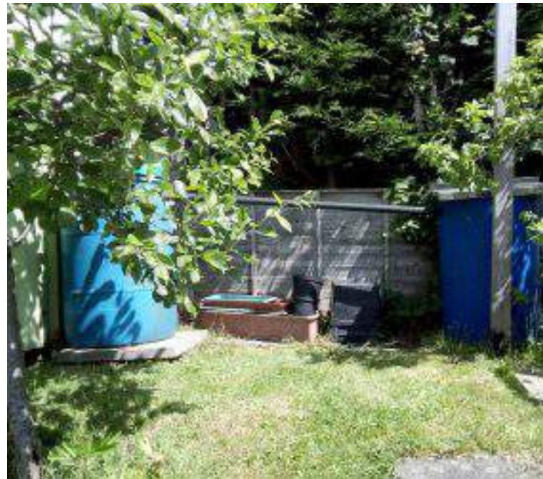
Fixed guttering on the shed to harvest any rainwater into two water butts.
